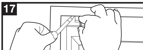
Position the slide stop (**F**) in the top screen door pocket just inside the far vertical stile on the inactive patio door panel and mark.
